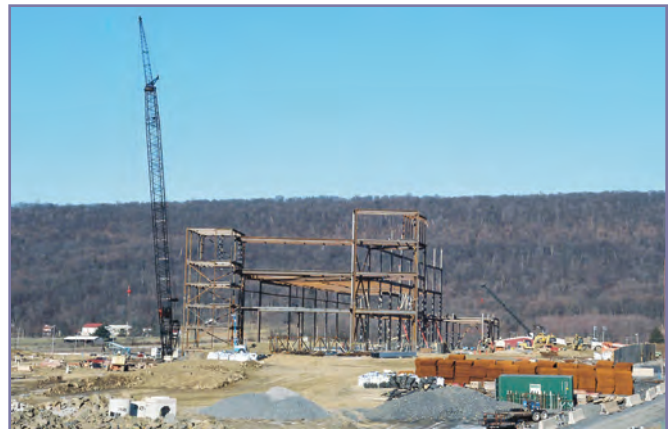
Penn National Construction Site
